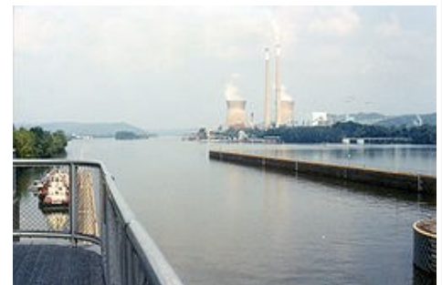
Pleasants power plant
