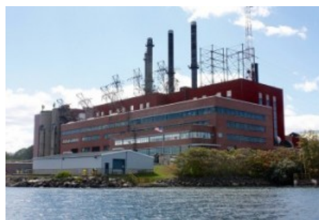
Schiller Station | Conservation Law Foundation
