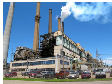
Conesville power plant | Ohio Citizen Action
