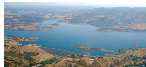
The 3-MW New Hogan Dam in Calaveras County, Calif. Small hydro facilities such as Hogan are automatically classified by CAISO as use-limited resources. | U.S. Army Corps of Engineers
