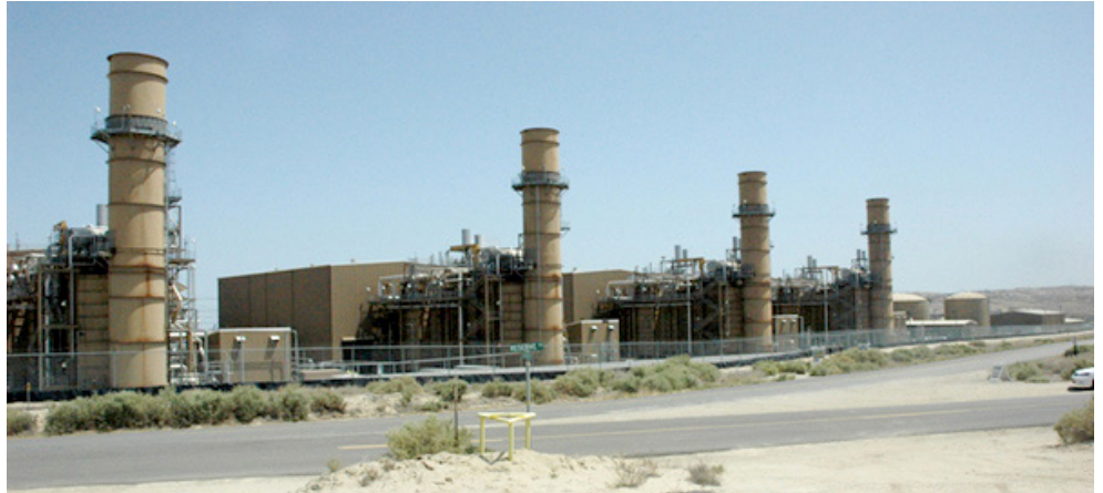
FERC denied a complaint by CXA La Paloma, owner of a natural gas plant in Kern County, alleging CAISO had facilitated an unjust market by failing to develop centralized capacity procurement. | Kern County, California Public Health Services Department
