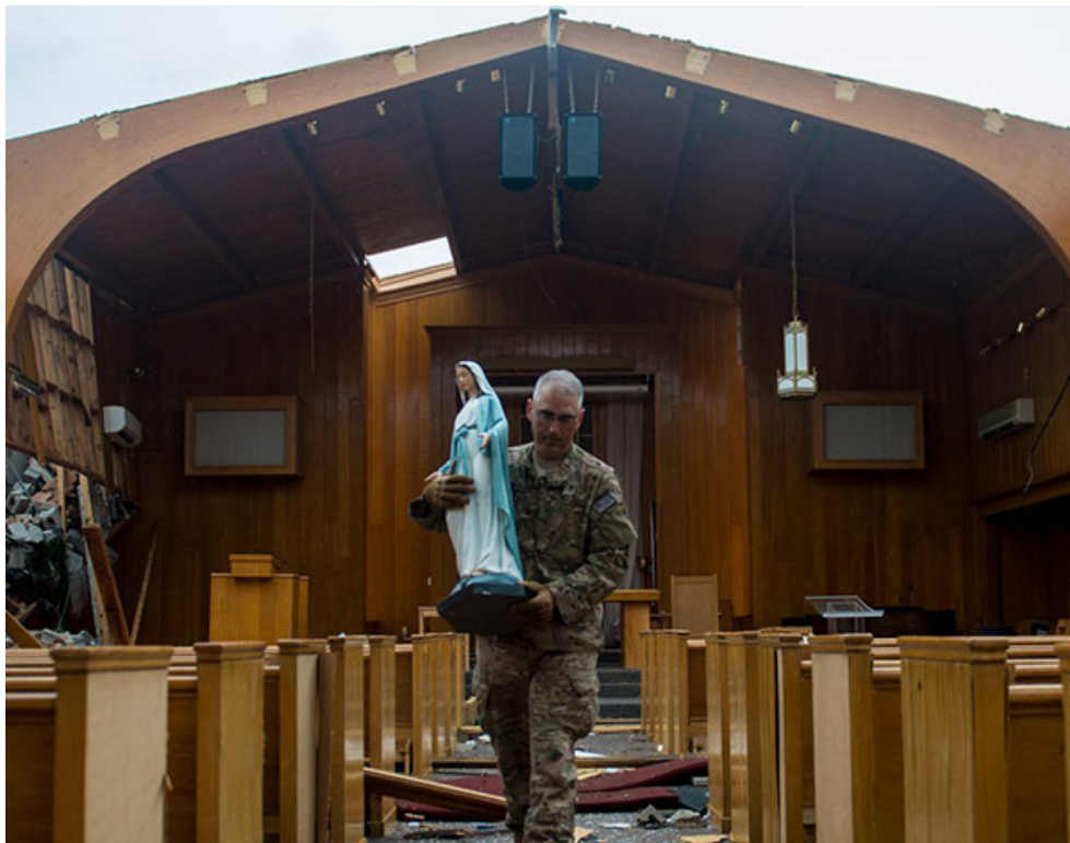
Hurricane Michael tore the roof off a chapel at Tyndall Air Force Base in Florida in October. | U.S. Air Force
