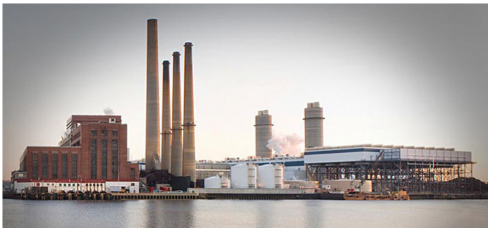
Mystic power plant
