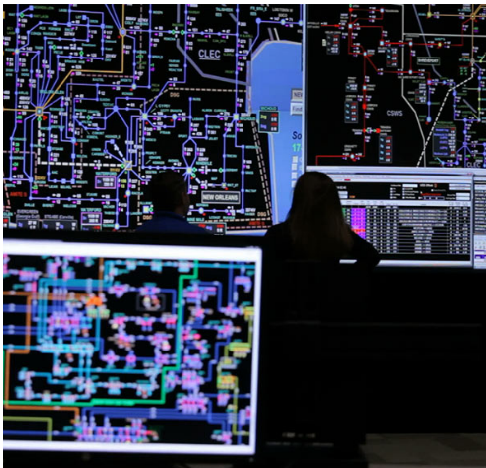
MISO control room | MISO
