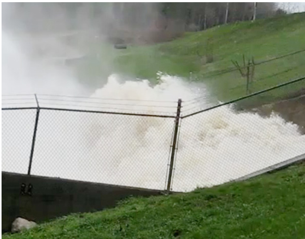
Edenville Dam spillway
