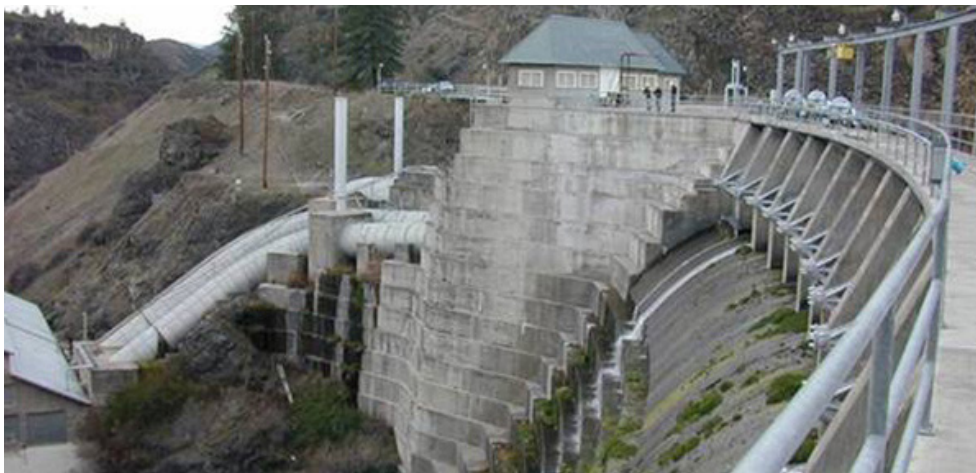
J.C. Boyle Dam and fish ladder, one of four Klamath dams slated for removal in 2020 | U.S. Fish and Wildlife Service
