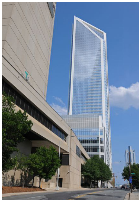
Duke Energy Center, Charlotte, N.C. | Duke Energy
