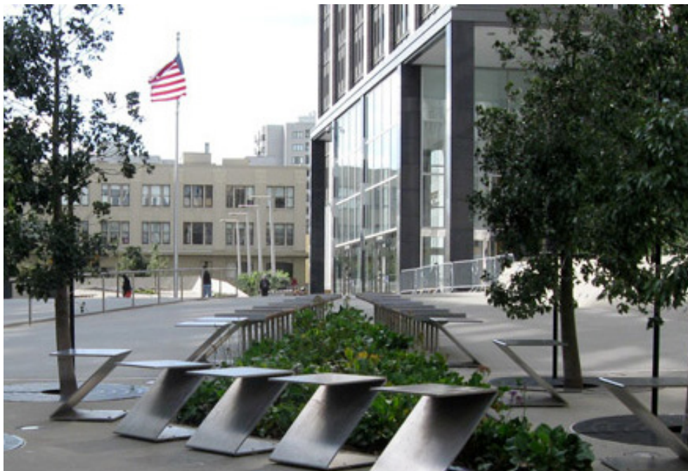
Philip Burton Federal Building, San Francisco | U.S. Bankruptcy Court - Northern District of California
