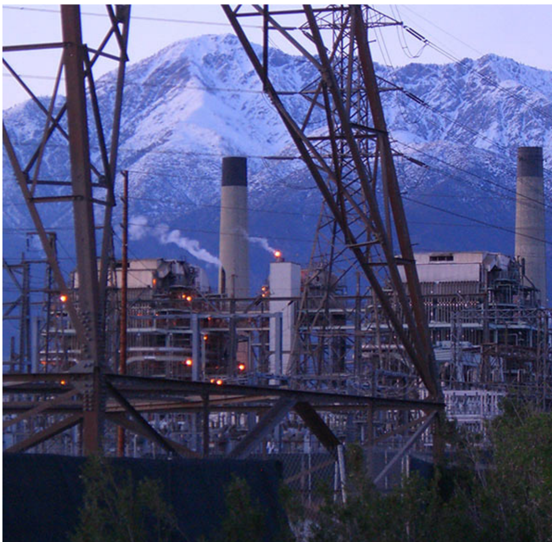
NRG's Etiwanda Generating Station
