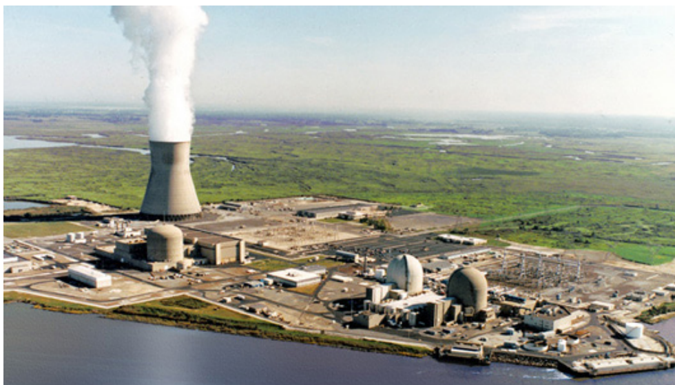
The Hope Creek and Salem nuclear units on Artificial Island in southern New Jersey | BHI Energy
