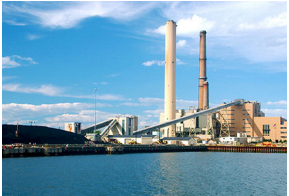
Salem Harbor Power Plant | Tetra Tech
