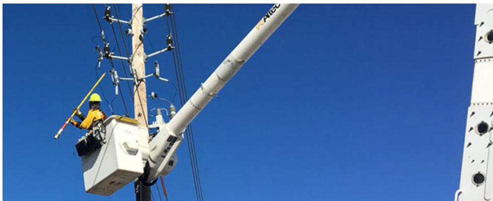
IPL crews restoring power Jan. 31 | Indianapolis Power and Light
