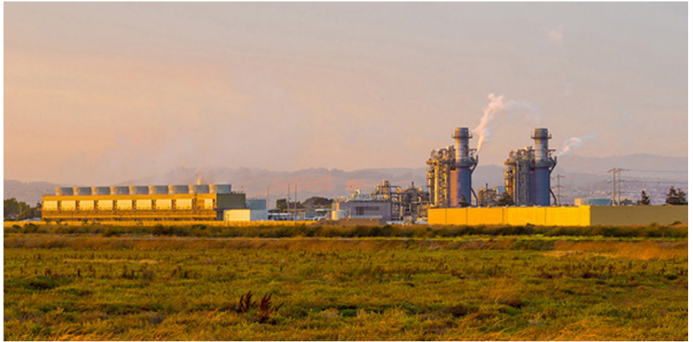
Calpine's Russell City Energy Center is one of the power plants at the center of the jurisdictional dispute between PG&E and FERC. | Calpine
