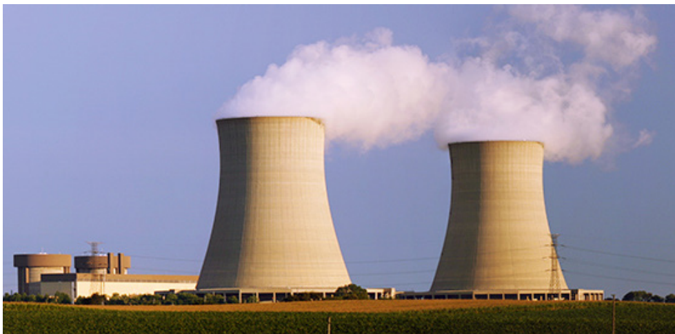
Exelon's Byron Generating Station's two nuclear reactors in Illinois produce more than 2,300 MW of electricity.
