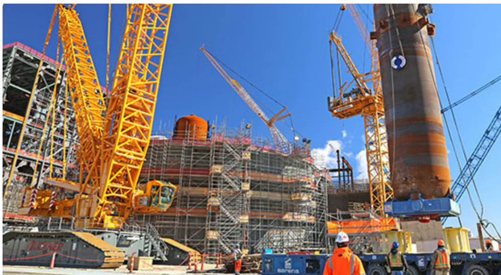
Vogtle nuclear plant construction | Georgia Power
