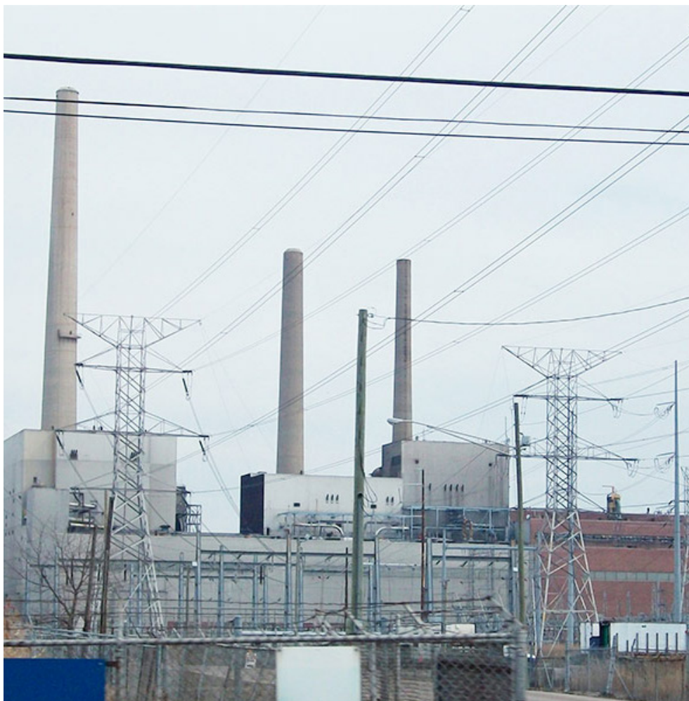
DTE Energy's St. Clair Power Plant is among coal plants that could close earlier than expected, exacerbating baseload generation retirements in MISO.
