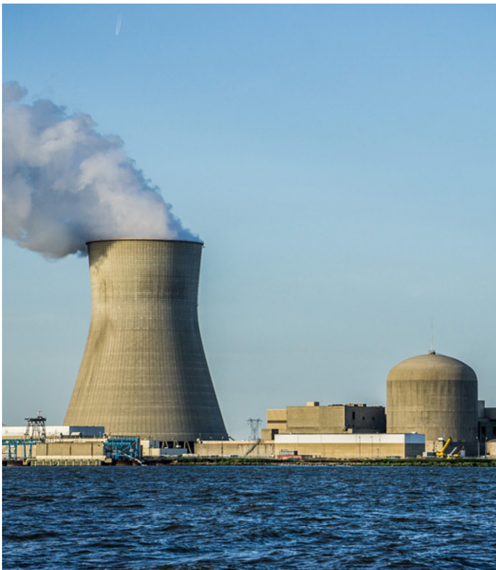
Hope Creek Nuclear Plant
