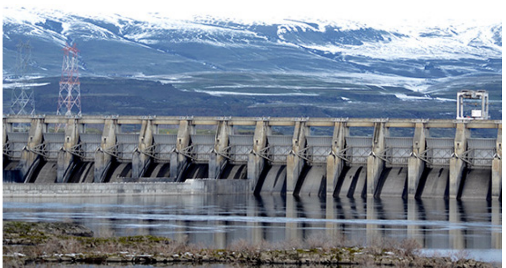
The Dalles Dam on the Columbia River is one of the major hydroelectric resources in Washington state. | © RTO Insider
