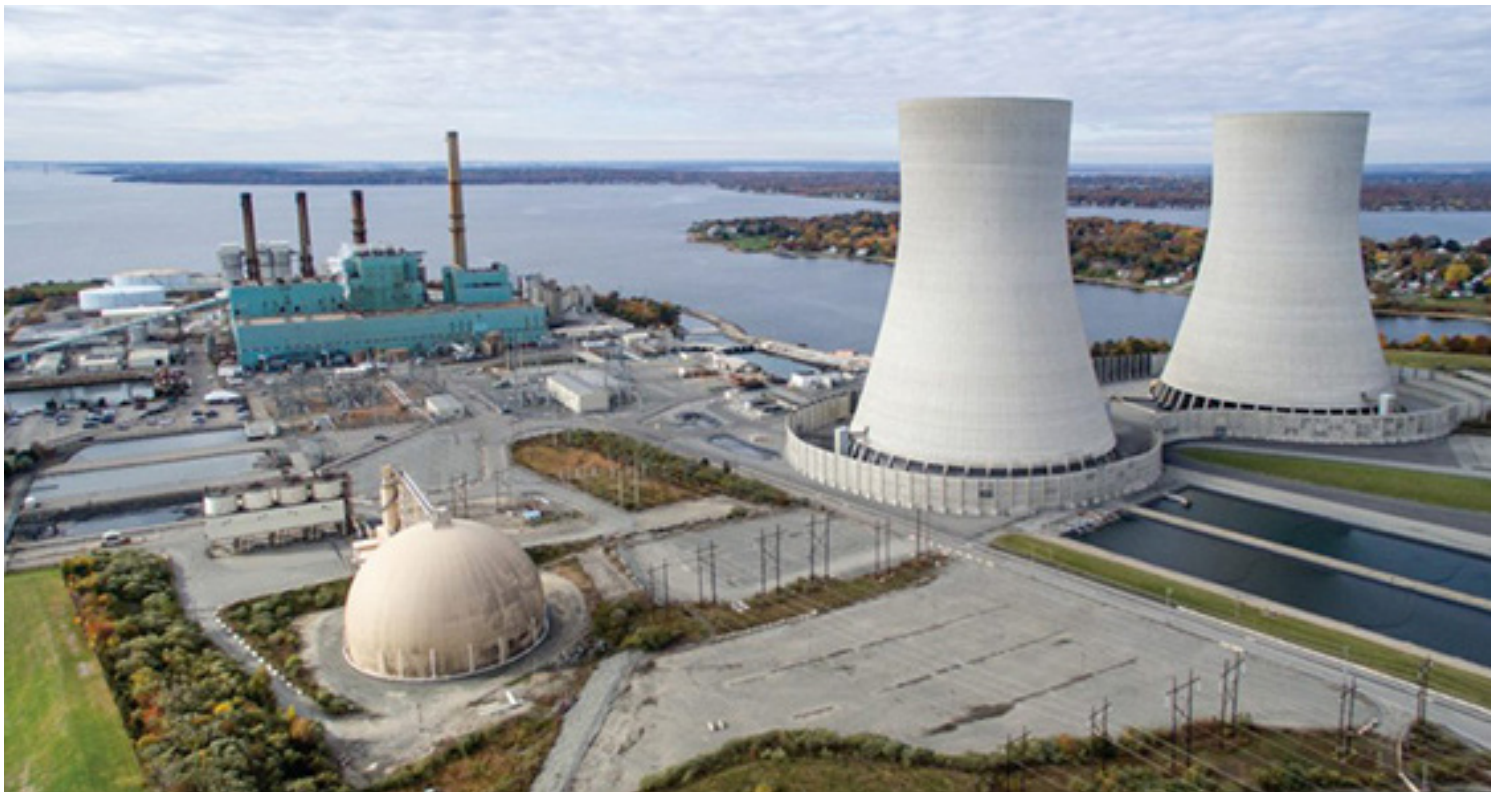
Brayton Point before the demolition of the cooling towers | Commercial Development Co.
