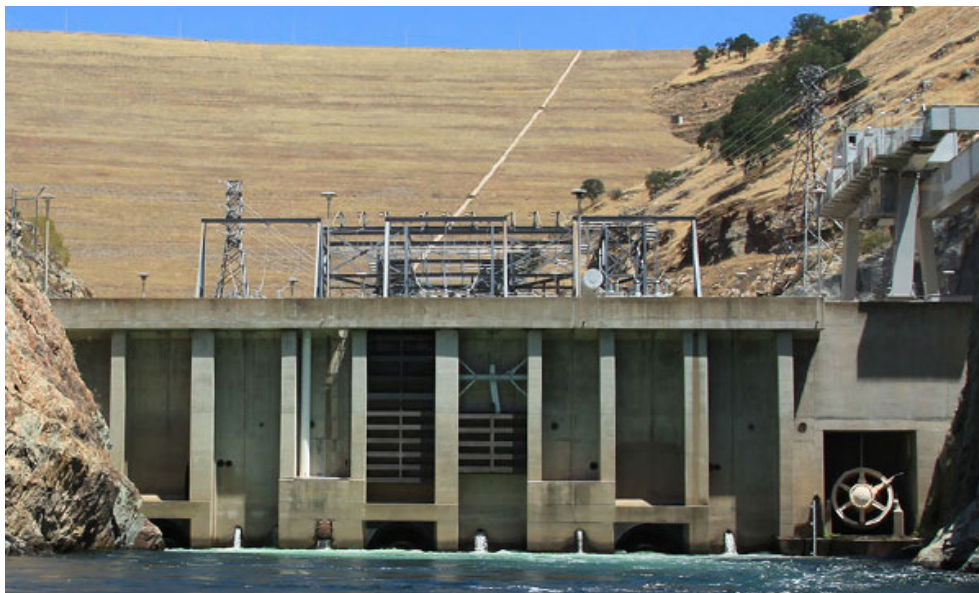
Turlock Irrigation District operates the 203-MW Don Pedro Dam in partnership with Modesto Irrigation District. | Turlock Irrigation District
