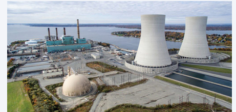
Brayton Point before the demolition of the cooling towers (p.13) | Commercial Development Co.
