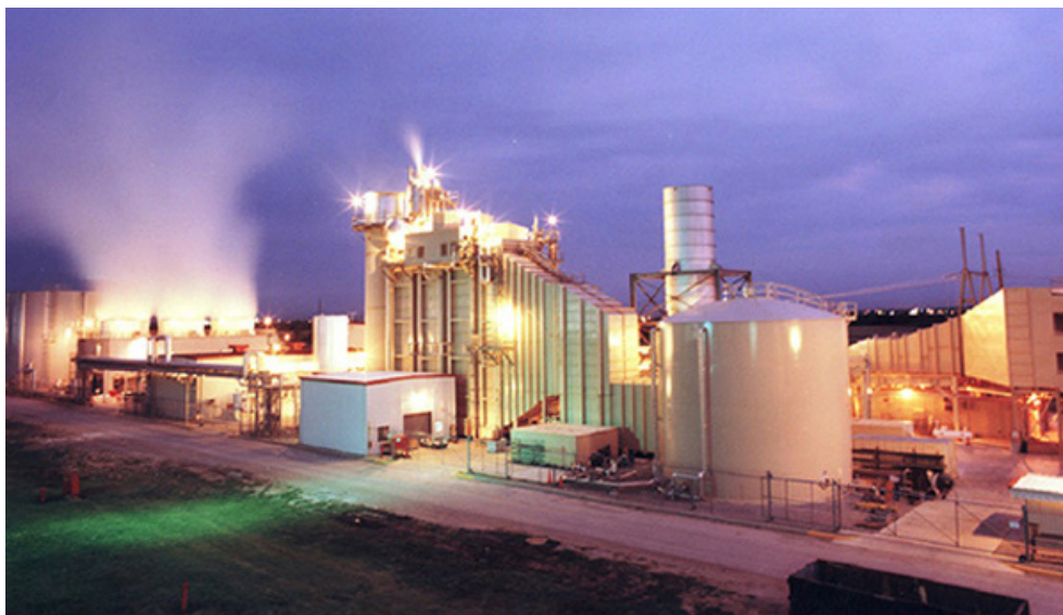
Oklahoma Cogeneration plant | Oklahoma Cogeneration
