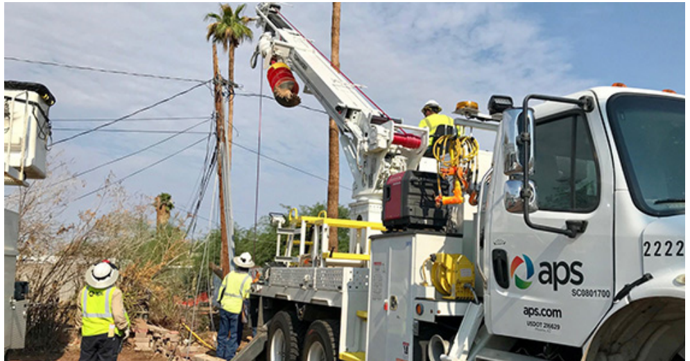
Arizona Public Service raised questions about how balancing authorities should react when their area control error (ACE) is at odds with an interconnection's frequency. | Arizona Public Service
