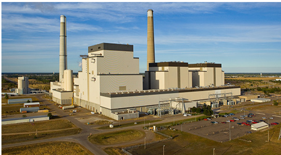
Sherco Generating Station | Xcel Energy
