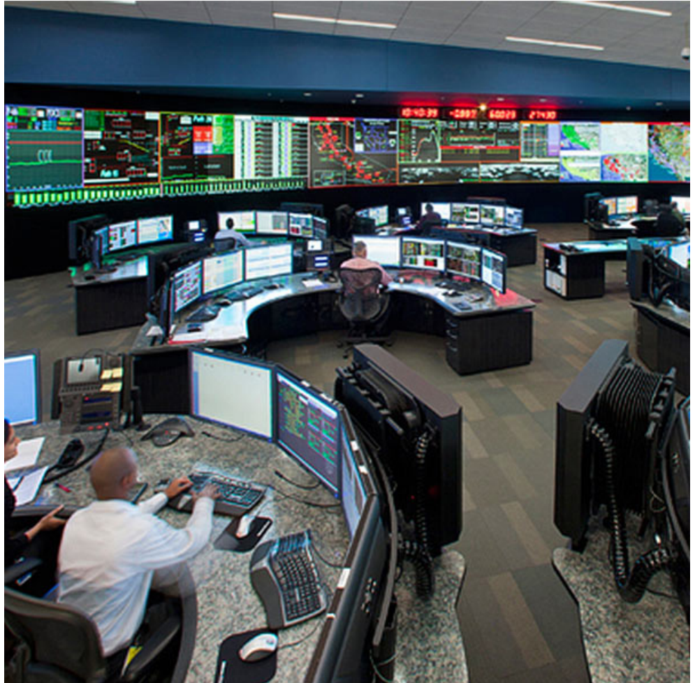
CAISO's control room in Folsom, Calif. | CAISO
