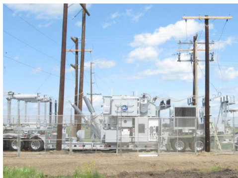
Delta Star, a Virginia-based provider of substation equipment, said FERC should encourage the use of trailer-mounted mobile substations. | Delta Star
