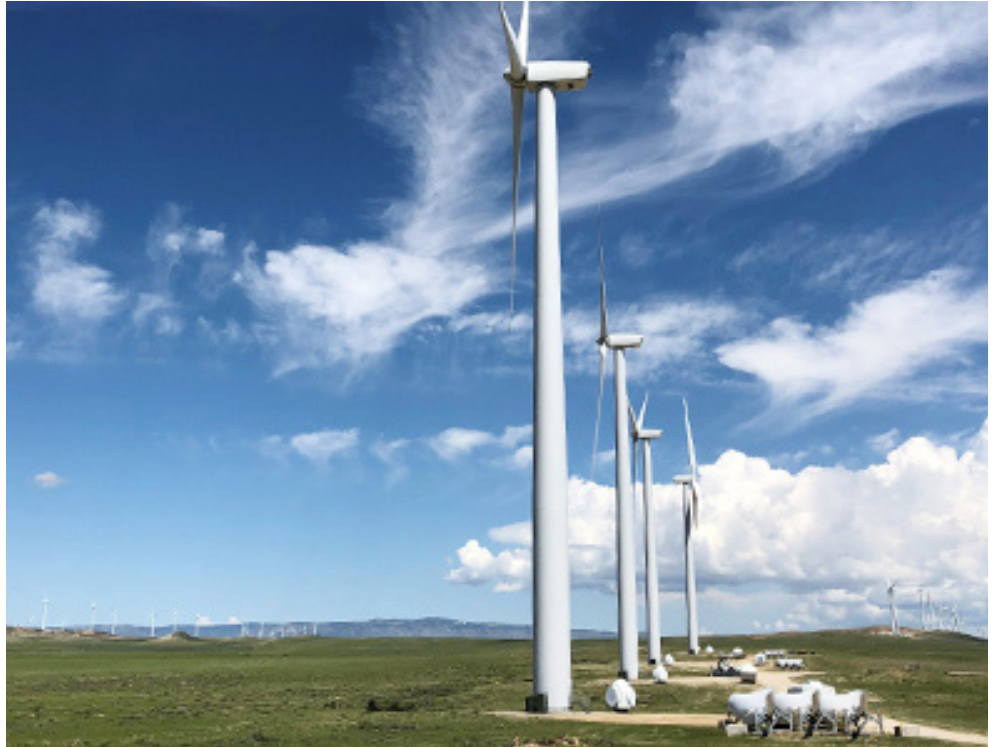
Rocky Mountain Power, a division of PacifiCorp, plans to add 1,150 MW of new wind power and a 140-mile high-voltage transmission line near its existing Seven Mile Hill wind farm in Carbon County, Wyo. | © RTO Insider
