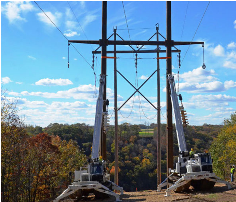
ITC Midwest builds a transmission line in Iowa in 2013. | ITC Midwest
