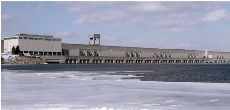
St. Lawrence-Franklin D. Roosevelt Power Project on the St. Lawrence River | NYPA
