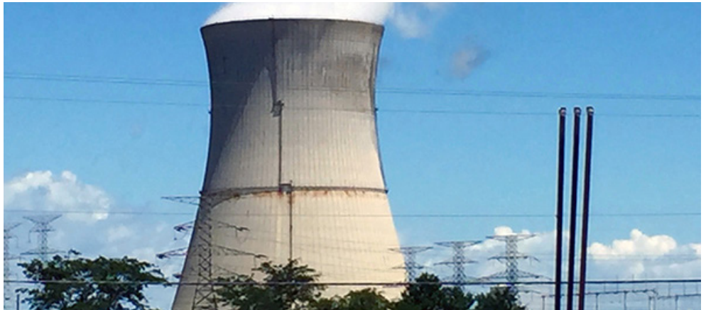
Davis-Besse Nuclear Power Plant
