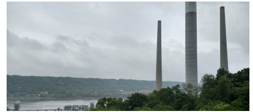
OVEC's Clifty Creek power plant
