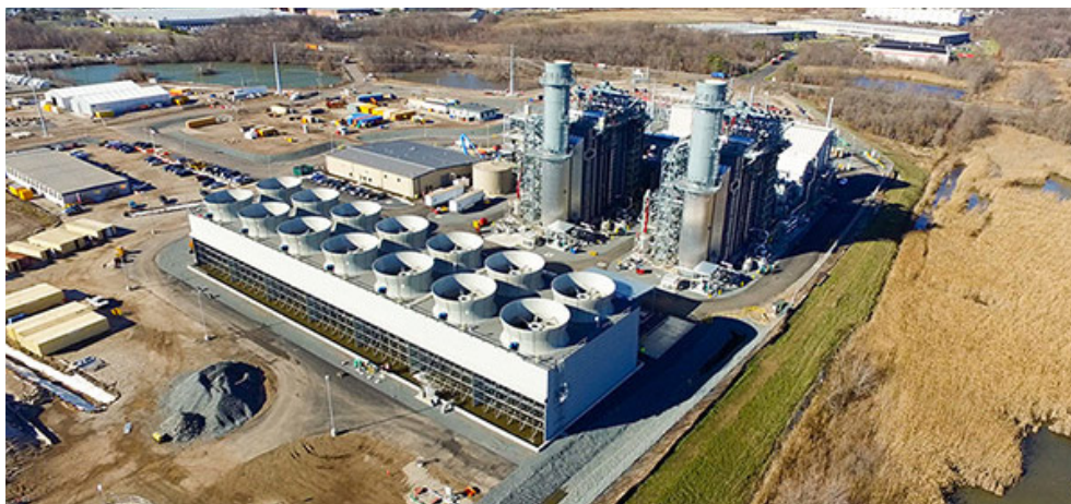
Competitive Power Ventures' Woodbridge Energy Center | Competitive Power Ventures
