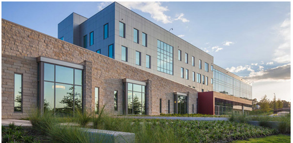
SPP's corporate campus | Nabholz Construction
