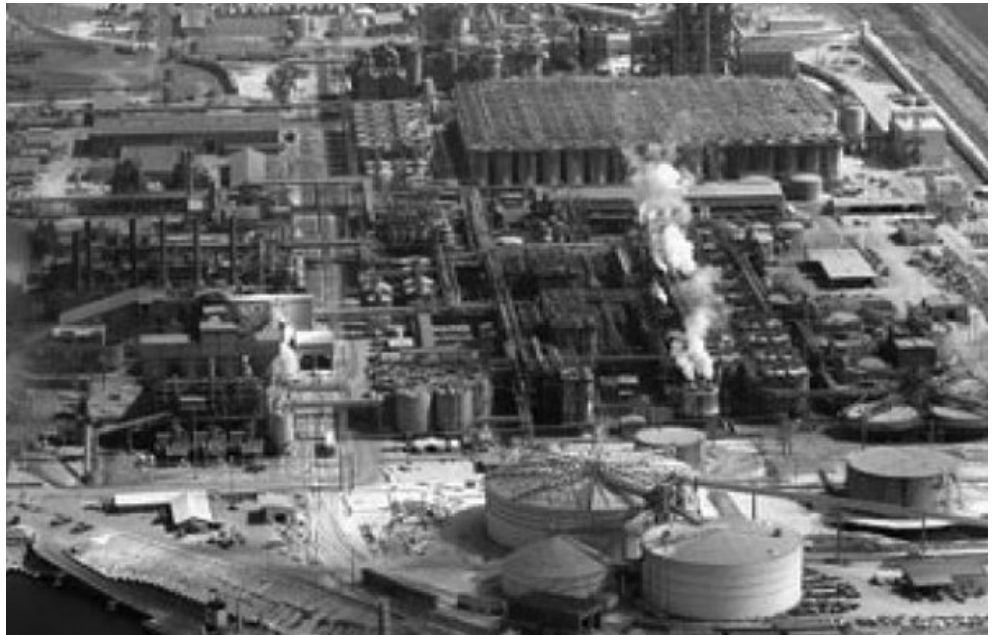
The Sherwin Alumina plant, Gregory Power Partners' cogeneration partner, shut down in 2016. | Sherwin Alumina
