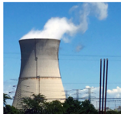
Davis-Besse nuclear power plant
