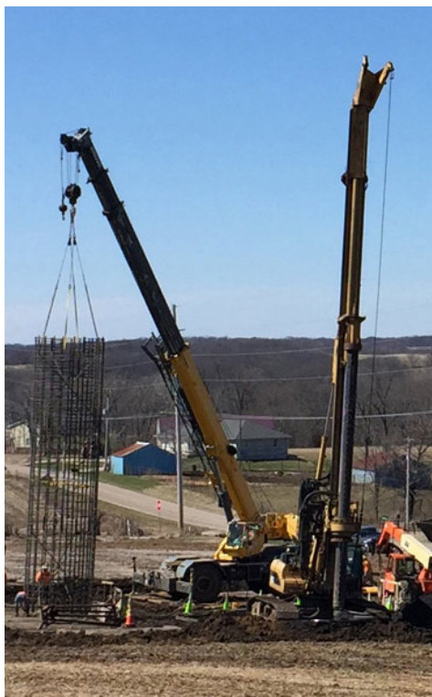
Construction of Ameren's Illinois Rivers transmission line | Plocher Construction
