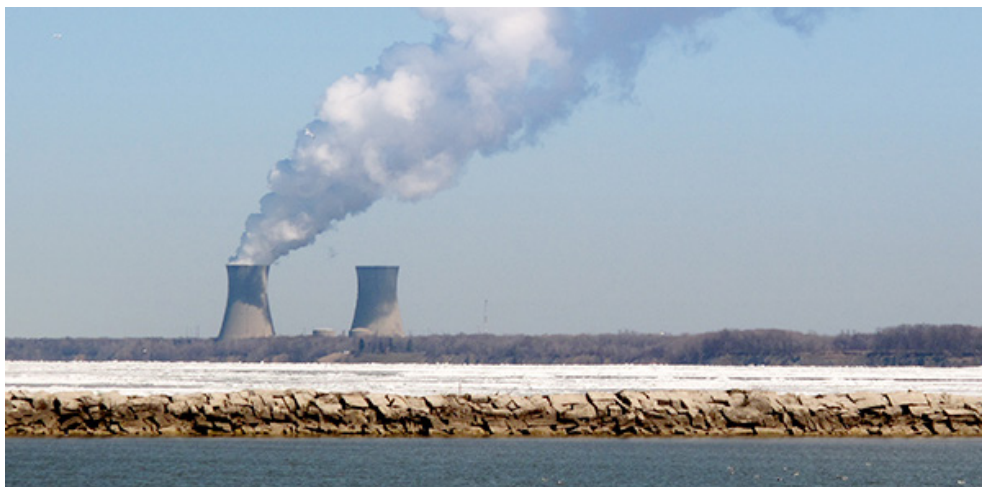
Perry Nuclear Power Plant, located about 40 miles northwest of Cleveland
