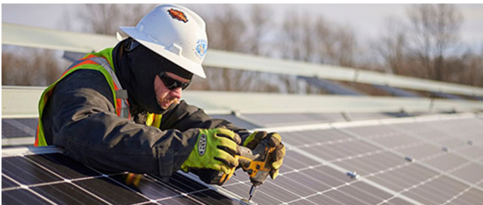
Solar panel construction | Consumers Energy
