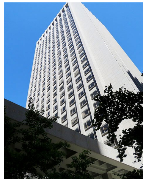
PG&E headquarters in San Francisco | © RTO Insider
