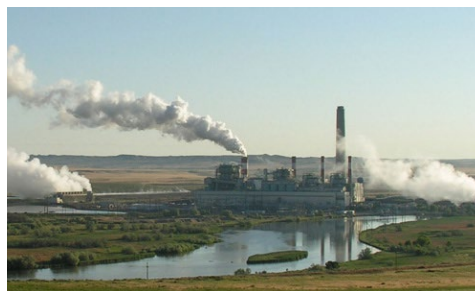
Dave Johnston coal-fired plant in Wyoming
