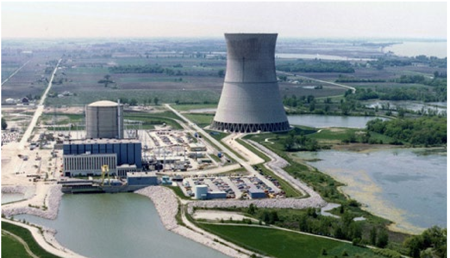
The Davis-Besse nuclear plant in northern Ohio | NRC
