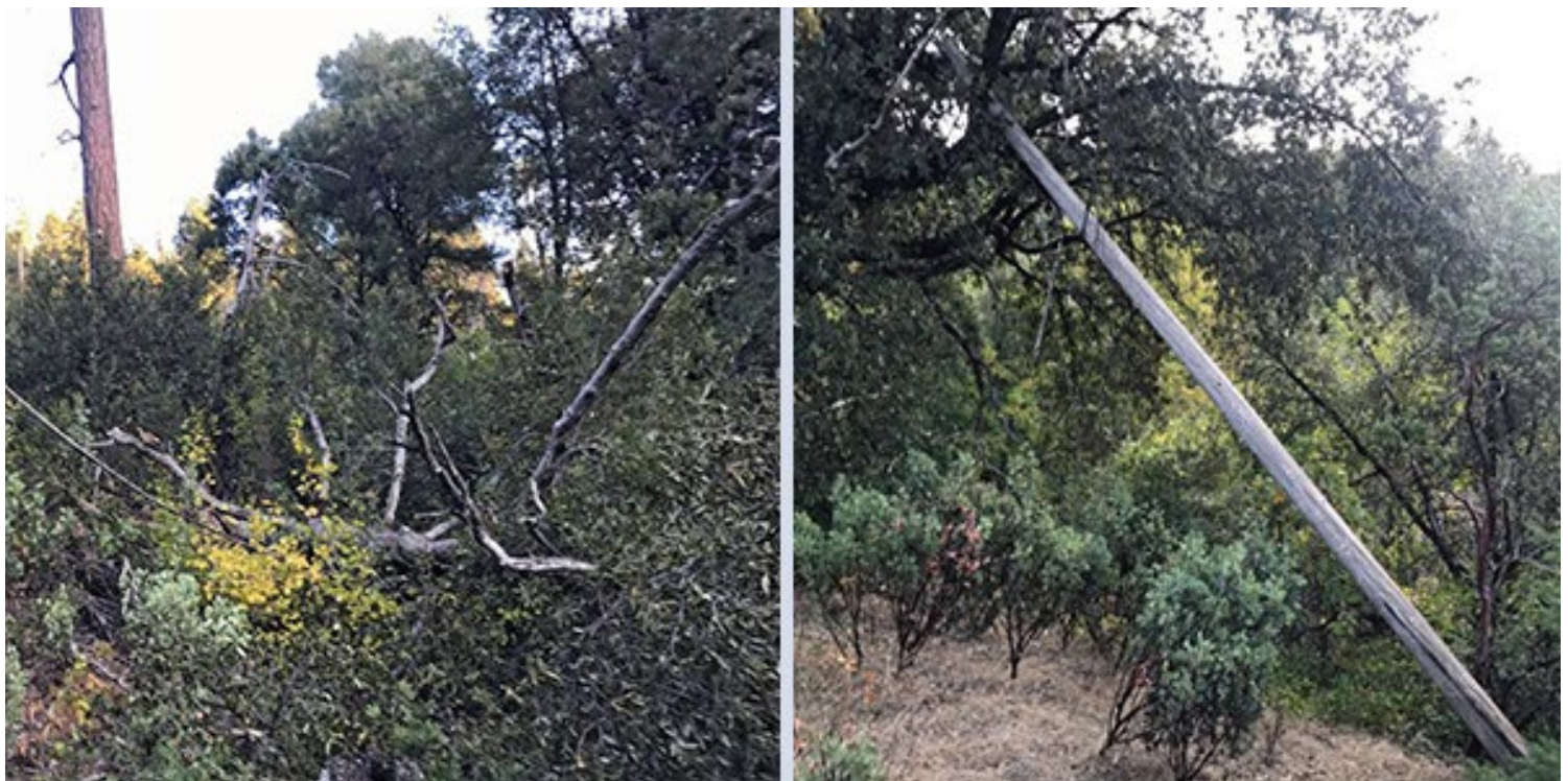
PG&E said it recorded about 100 instances of damage to its equipment in areas affected by its PSPS, including these downed lines in Shasta County. | PG&E
