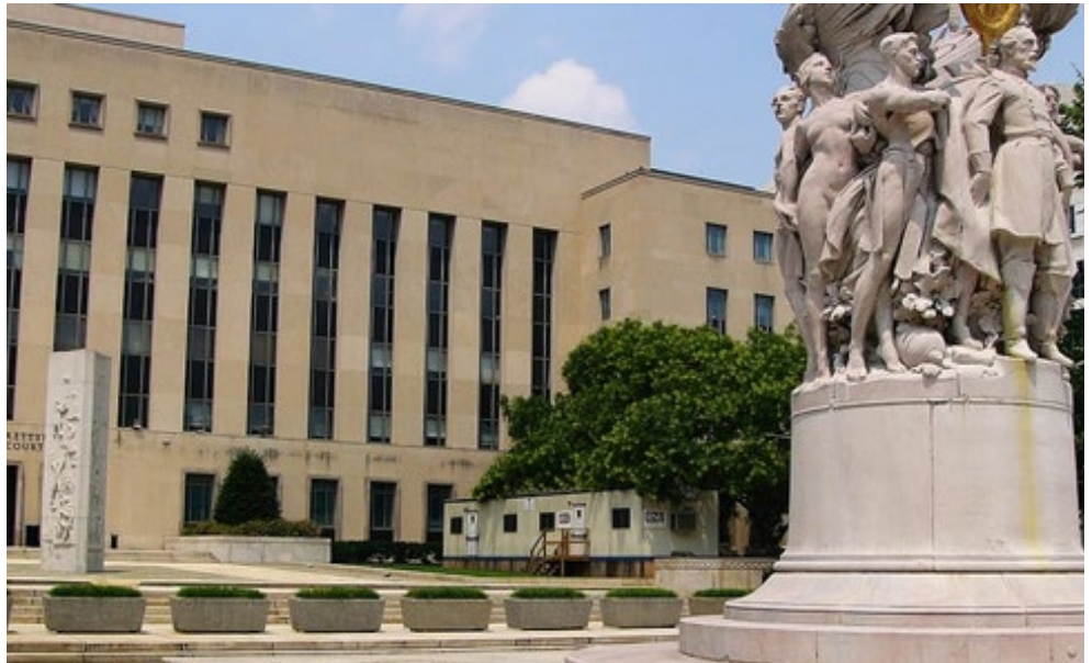
E. Barrett Prettyman Federal Courthouse | HSU Builders
