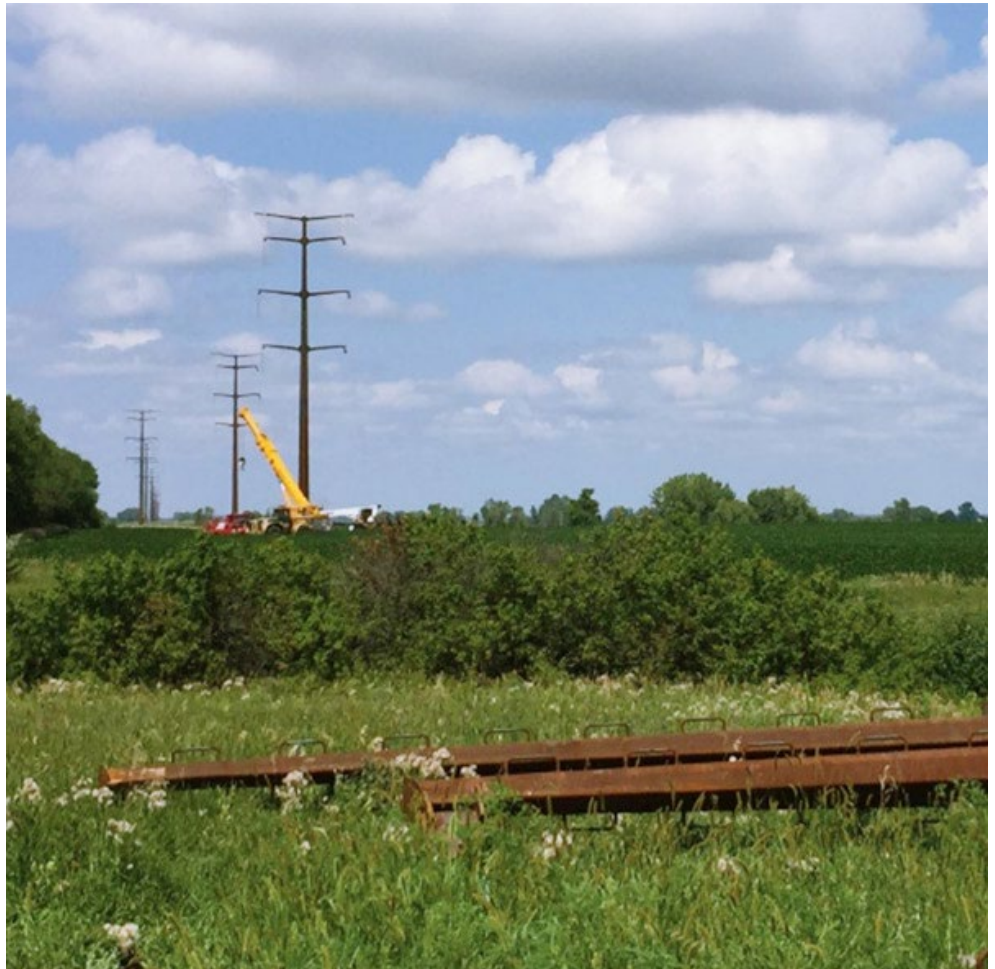
CapX2020 construction | CapX2020
