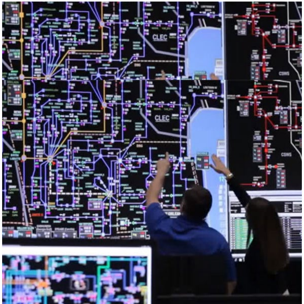
MISO control room. | MISO
