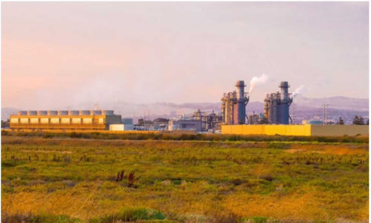
Calpine's Russell City Energy Center in Hayward, Calif. | © RTO Insider
