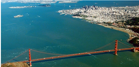
The Trans Bay Cable runs for 53 miles under San Francisco Bay. | © RTO Insider
