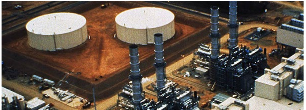
The Doswell Energy Center in Hanover County, Va. | Fluor
