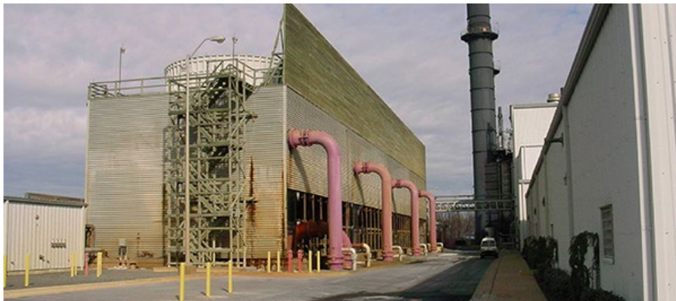
The Brandywine Power Facility in Prince George's County, Md. | Brandywine Power
