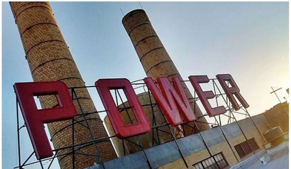
EPE's Rio Grande Plant in Sunland Park, N.M. | El Paso Electric
