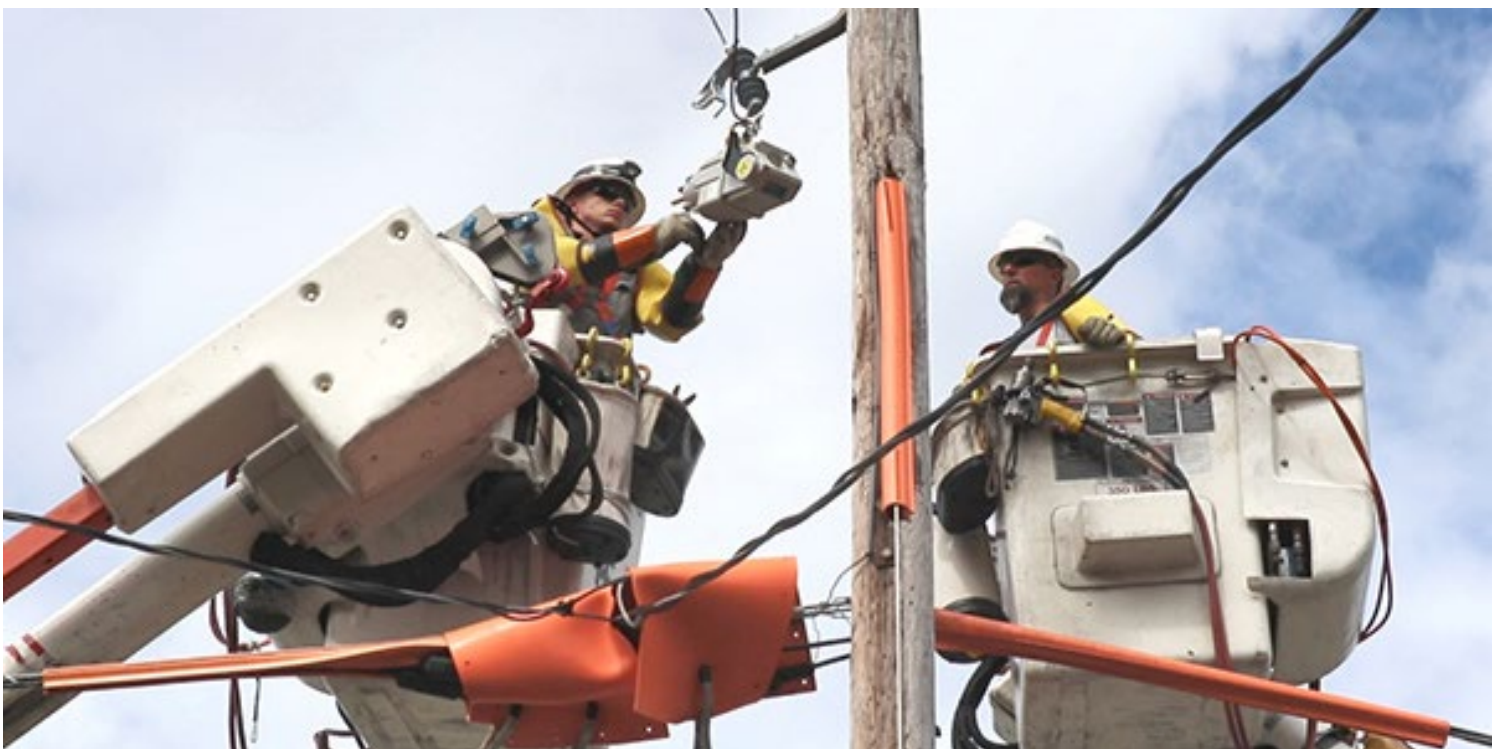
JCP&L linemen at work | FirstEnergy
