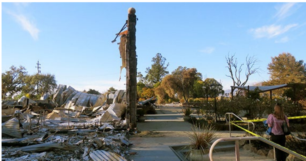
The stone facade was all that remained standing of the Soda Rock Winery days after the Kincade Fire tore through Sonoma County. | © RTO Insider
