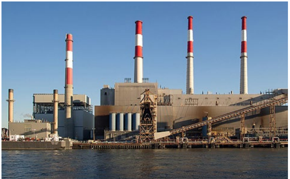
Ravenswood Generating Station
