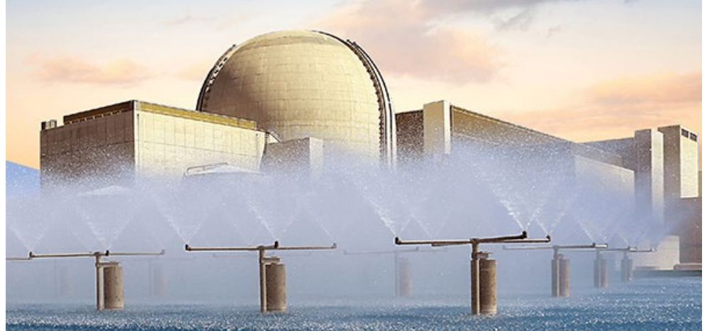
Arizona Public Service operates the Palo Verde Generating Station near Phoenix. | APS
