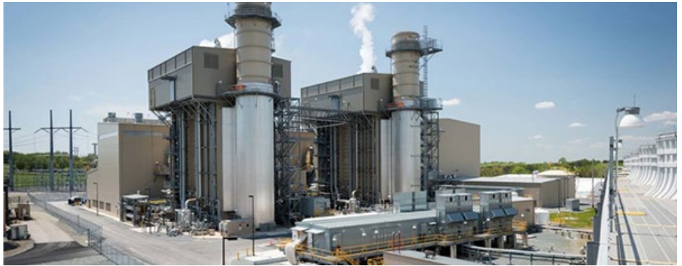
Old Dominion Electric Cooperative added the 1,000-MW Wildcat Point combined cycle plant less than two years ago. ODEC fears it may be the last capacity it can add under FERC's Dec. 19 decision to subject new self-supply units to the minimum offer price rule. | Old Dominion Electric Cooperative
