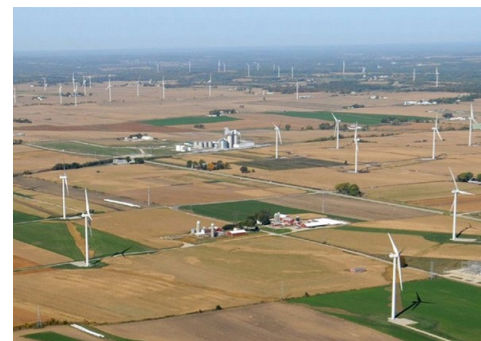
We Energies' Glacier Hills Wind Park | WEC Energy Group
