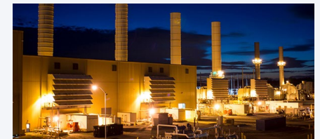
East Kentucky Power Cooperative's Bluegrass Station in LaGrange, Ky. | East Kentucky Power Cooperative
