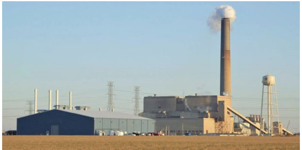
Merom Generating Station | Hoosier Energy
