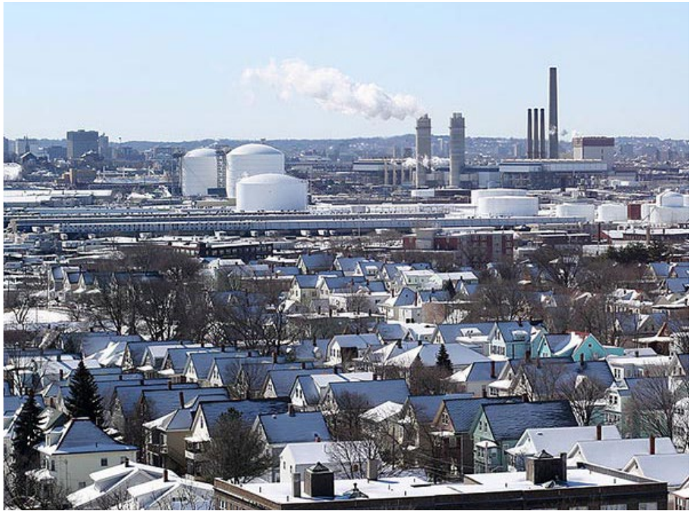
Everett, Mass., with Exelon's Mystic Generating Station in the background
