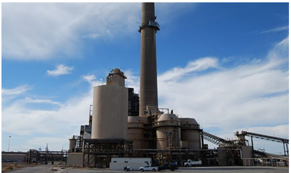
Oklaunion Power Station | AEP
