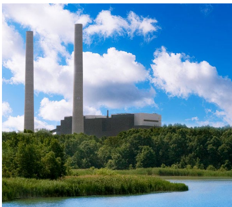
DTE's Belle River power plant | DTE Energy
