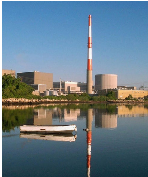
Dominion is replacing the Millstone Unit 3 generator and feedwater measurement equipment, which will bump the unit's year-round output to 1,262 MW, just over ISO-NE's interconnection limit for such resources. | NRC
