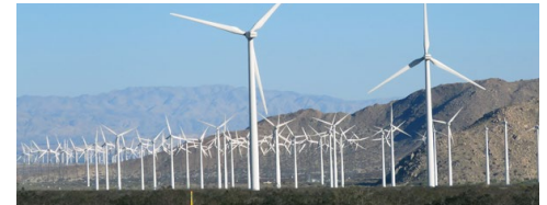
Wind farm near Palm Springs | © RTO Insider
