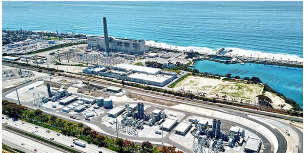
NRG's Encina Power Station near San Diego | NRG
