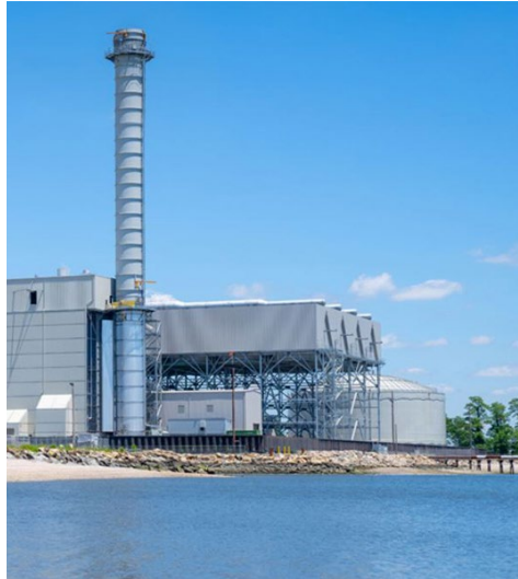
Bridgeport Harbor 5, a 485-MW combined cycle plant in Connecticut that began operating last year, is PSEG's largest generating unit in New England. | PSEG
