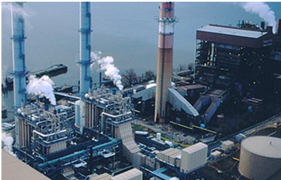
Dominion's 1,661-MW Possum Point Power Station in Dumfries, Va., can burn natural gas and oil. | © RTO Insider
