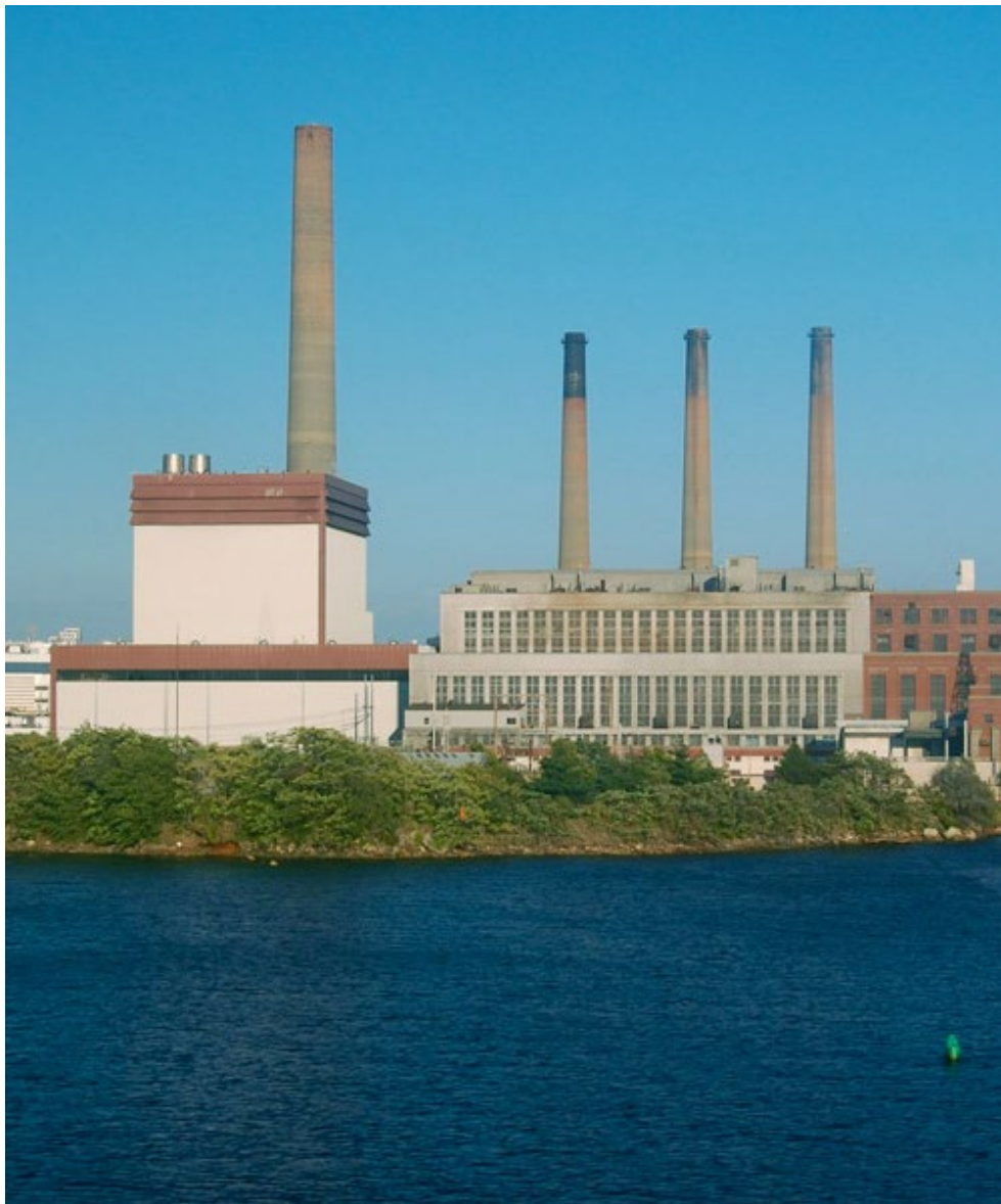
Mystic Generating Station, on the Mystic River in Everett, Mass.
