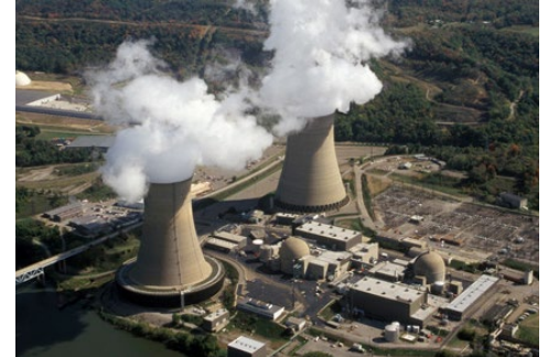
Beaver Valley Nuclear Power Plant
