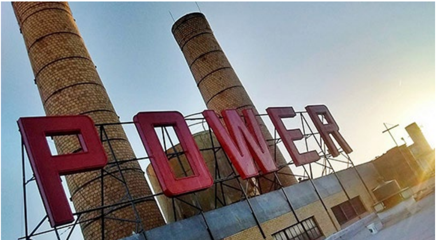
EPE's Rio Grande Plant in Sunland Park, N.M. | El Paso Electric
