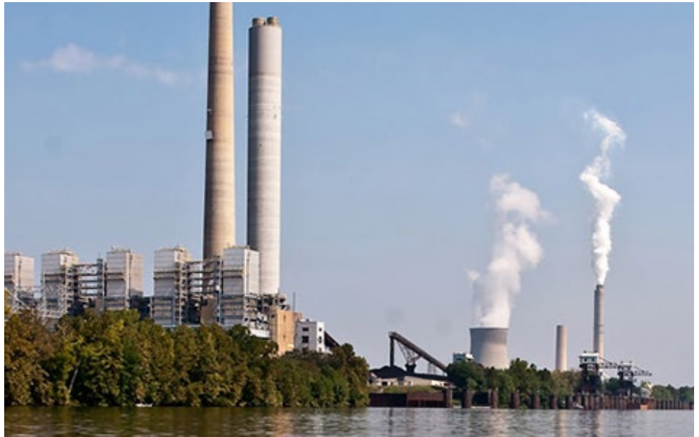
Kyger Creek Power Plant
