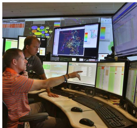
Inside SPP's control room | SPP
