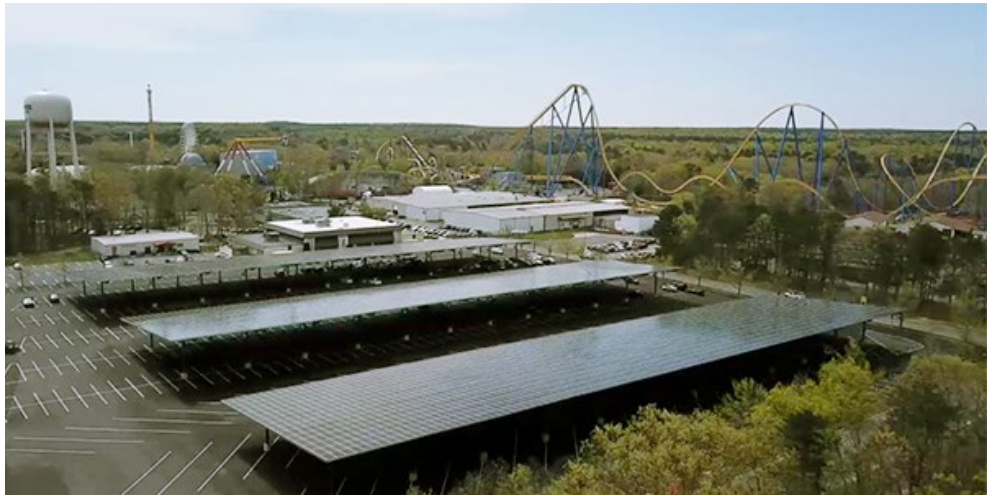
The Six Flags Great Adventure amusement park in Jackson, N.J., is mostly powered by a 23.5-MW solar project that began operation last summer. | Six Flags
