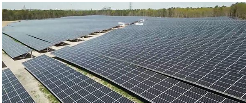
Six Flags said its array — 11 MW of solar carports and 12.5 MW on 40 acres of ground-mounted solar panels — makes it New Jersey's largest net metered solar project. | Six Flags
