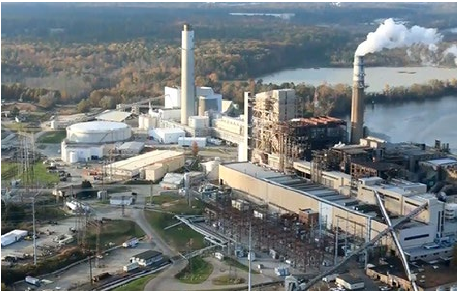
Dominion Virginia Power's Chesterfield Power Station, which can produce 1,415 MW, has two coal-fired units and two combined cycle units. | Dominion Energy
