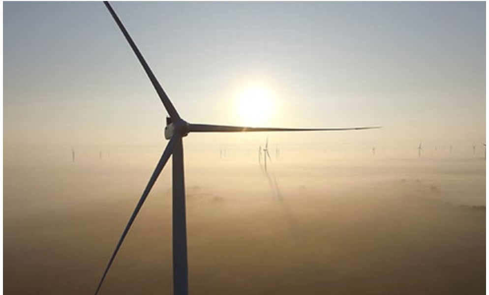
Radford's Run Wind Farm | E.ON
