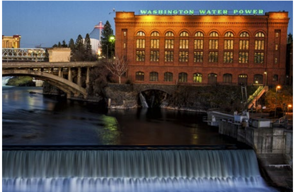
NWPP member Avista Utilities, formerly Washington Water Power, owns the Monroe Street hydroelectric plant in downtown Spokane. | Visit Spokane
