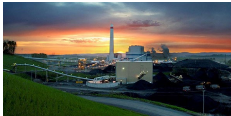
Longview Power plant near Morgantown, W.Va. | Longview
