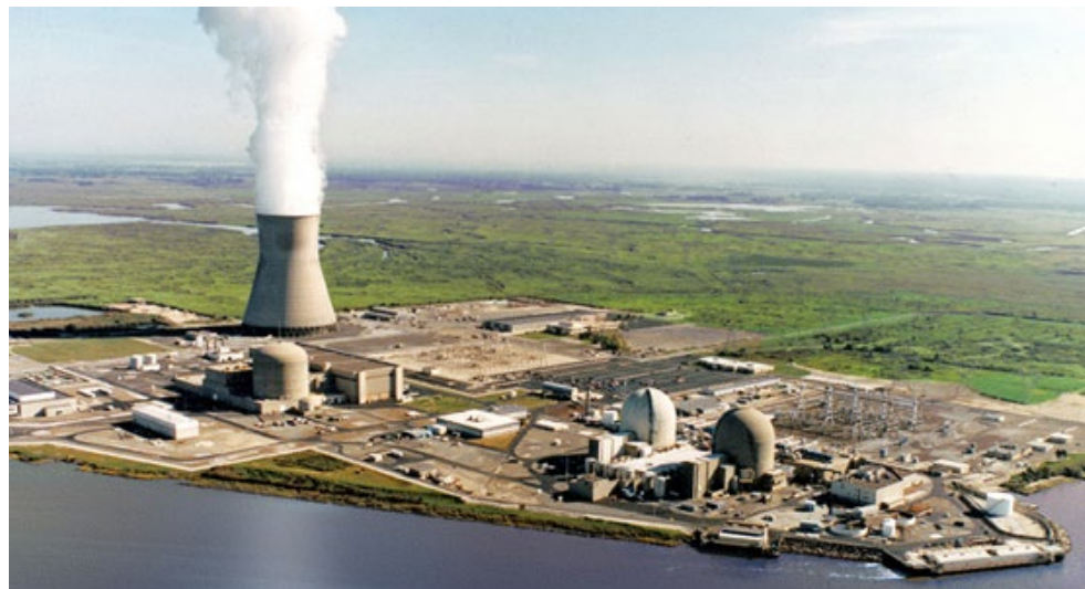
The Hope Creek and Salem nuclear units on Artificial Island in southern New Jersey | BHI Energy
