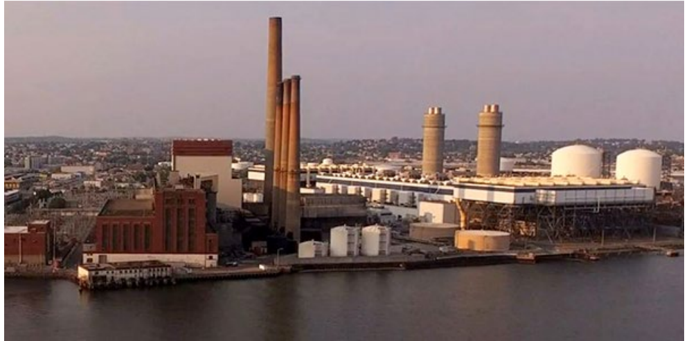
ISO-NE has kept Exelon's Mystic Generating Station operating under an expensive and controversial out-of-market contract for reliability reasons. | Anbaric Development Partners
