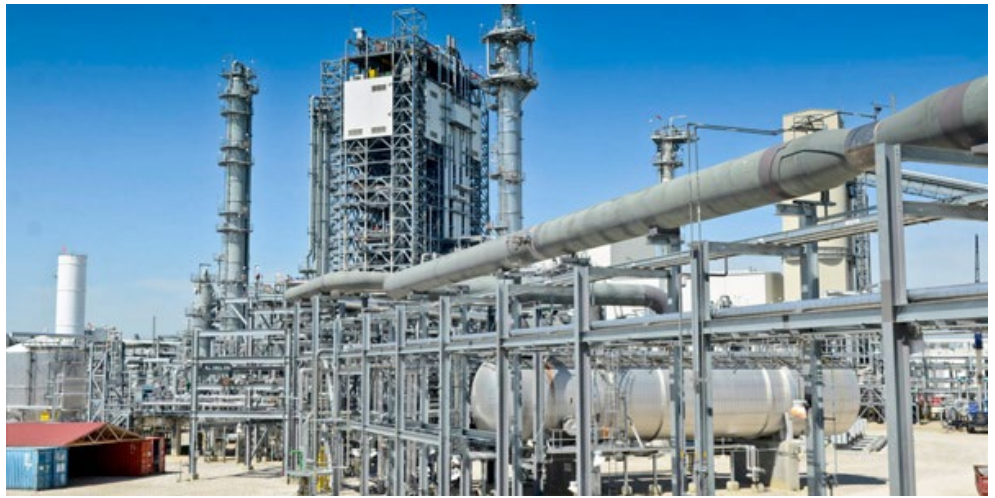
Edwardsport Integrated Gasification Combined Cycle plant | Duke Energy
