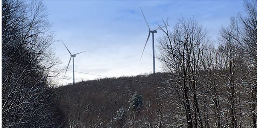
Wind farm near Altoona, Pa. | © RTO Insider
