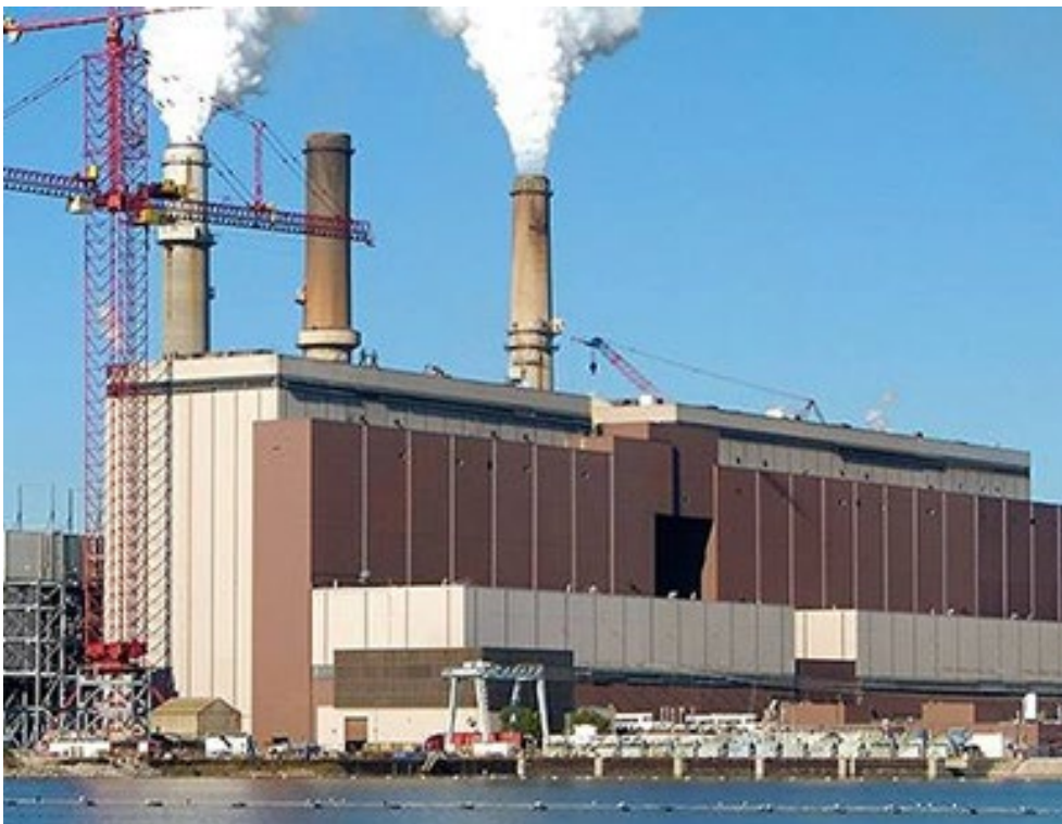
Gibson Generating Station | Duke Energy
