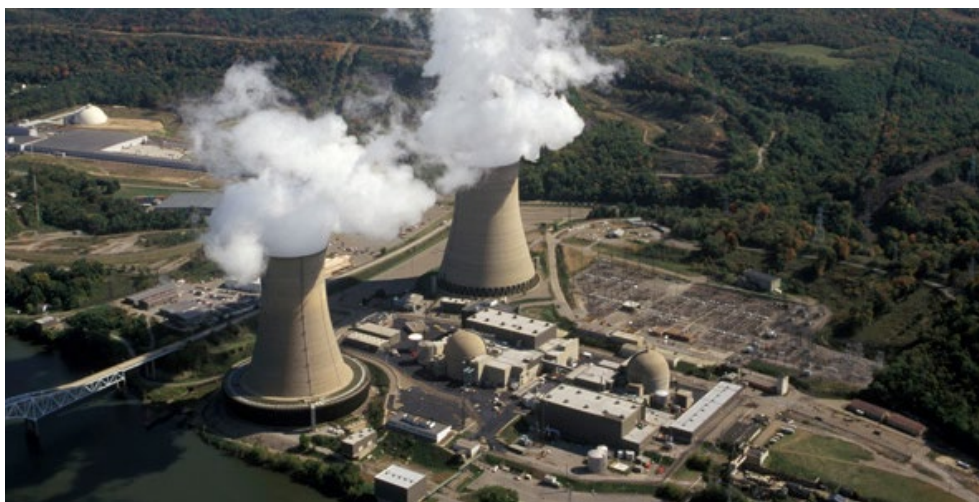
Beaver Valley Nuclear Power Plant
