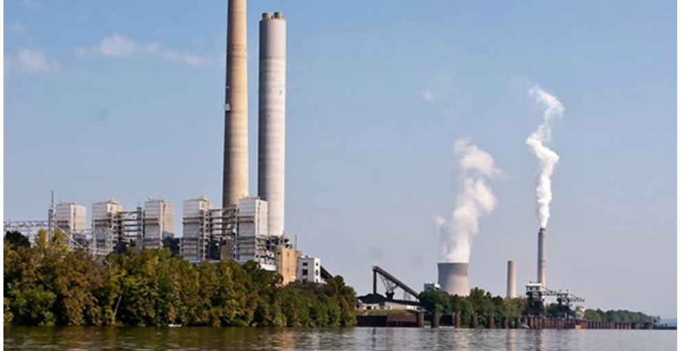
Ohio Valley Electric Corp.'s Kyger Creek Power Plant, a 1.08-GW coal-fired generator south of Cheshire, Ohio
