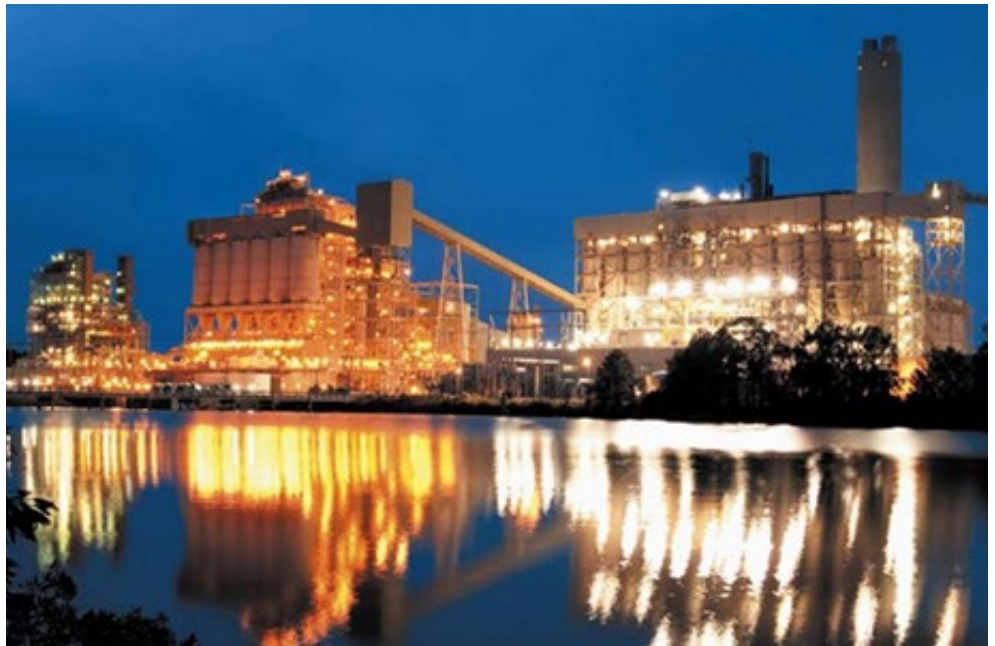
Dolet Hills power plant | Cleco Power
