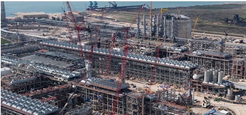
Cheniere's Corpus Christi LNG plant under construction | Cheniere Energy
