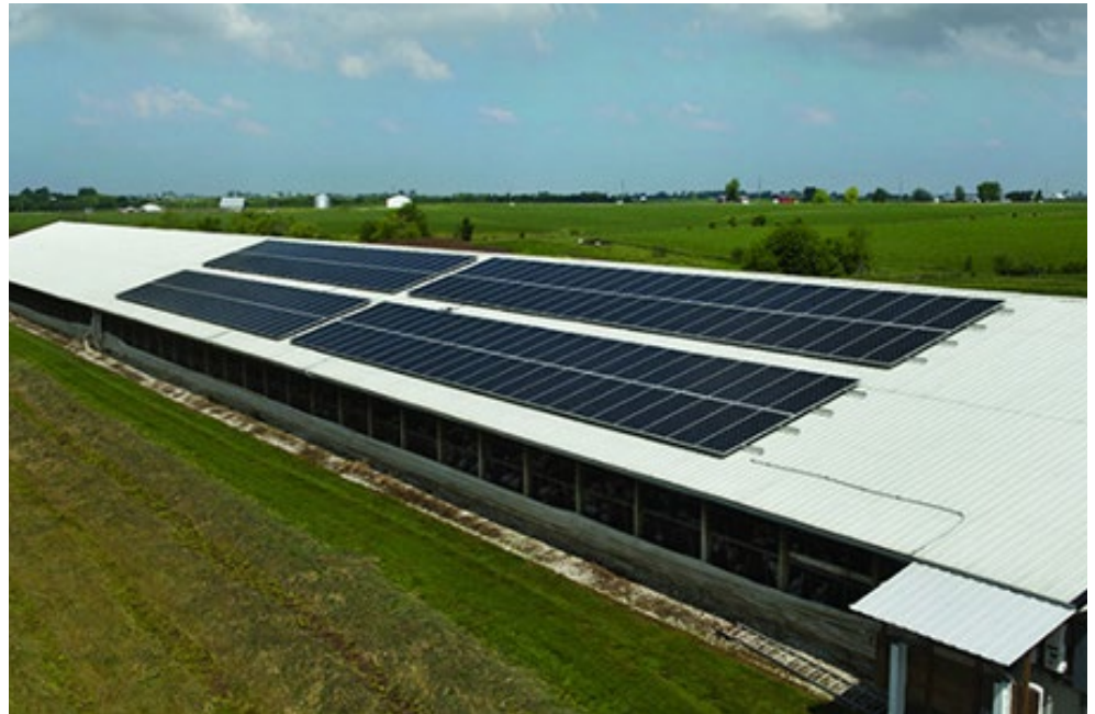
Solar panels line the roof of a turkey barn in Iowa. | Iowa Farm Bureau
