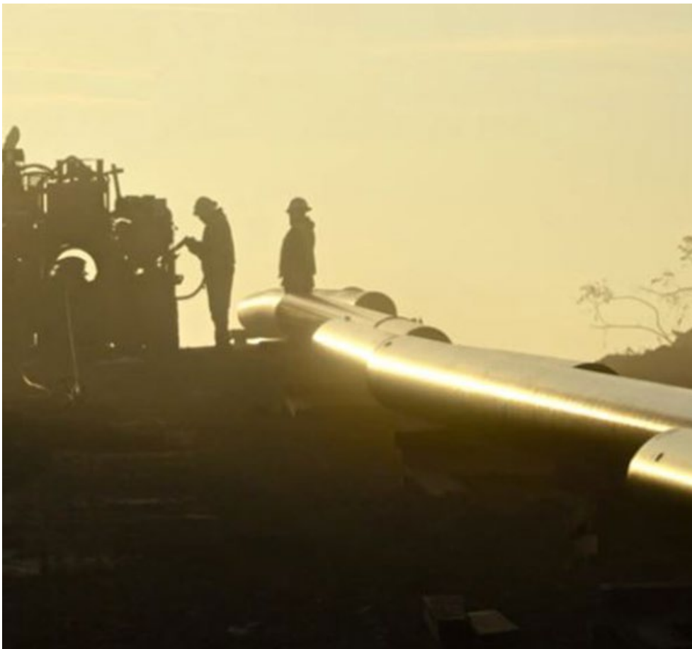
Natural gas pipeline construction | Williams
