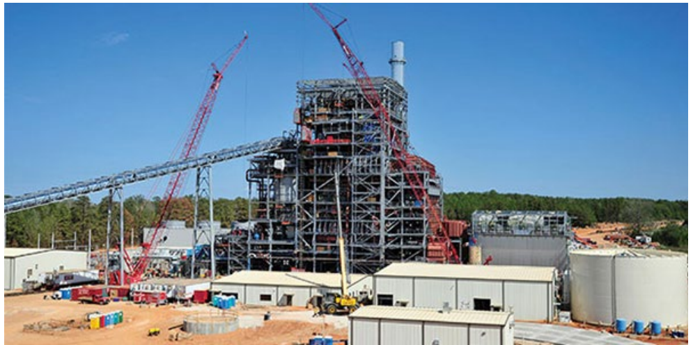
The Nacogdoches Generating Facility during its construction | Southern Co.
