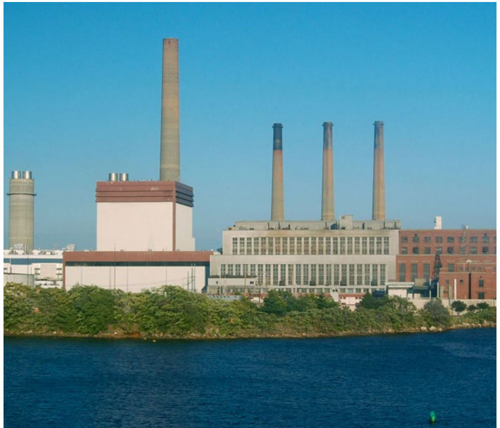
Mystic Generating Station, on the Mystic River in Everett, Mass.
