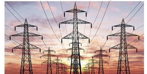
Long-haul transmission lines are key to the Macro Grid Initiative. (p.4) | Southwire
